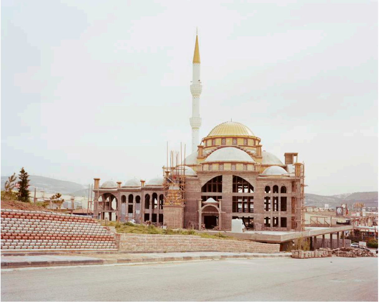
NORMAN BEHRENDT İVEDİK YAVUZ SULTAN SELİM CAMI, UNDER CONSTRUCTION, YENİMAHALLE, ANKARA 2016, FROM THE BRAVE NEW TURKEY SERIES.
